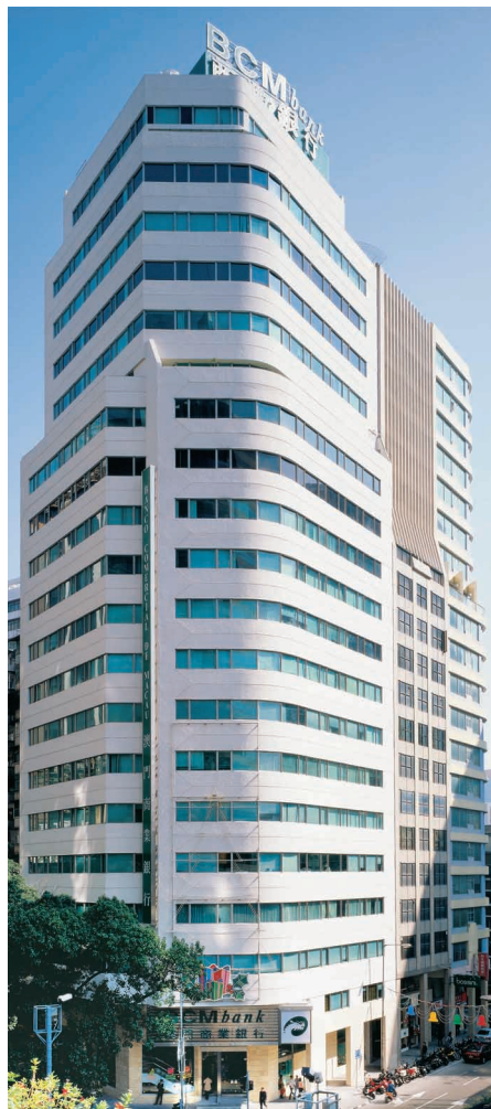
The Banco Comercial de Macau, S.A. headquarters building is located in the central business district of Macau. 澳門商業銀行總部大廈座落澳門主要商業中心樞紐。
